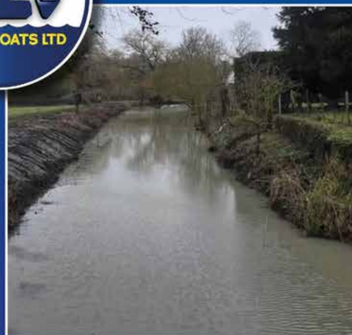
AFTER reed removal
